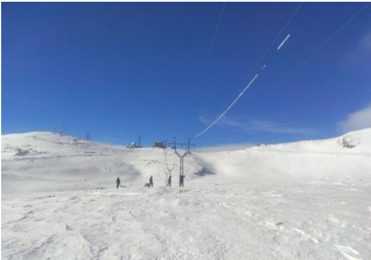
Figure 2. The sunny day helped us finish the repairs during the day.
