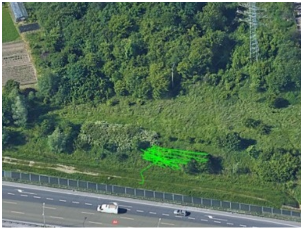
Fig. 5: Drone path view (green) under power line. A high voltage electric pole is visible in the right-top corner.
