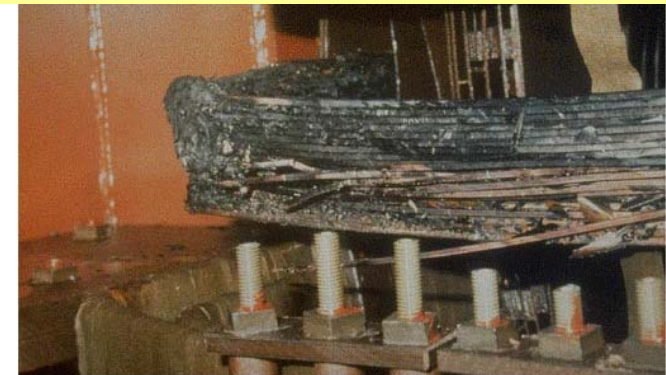
Damaged transformer windings.
