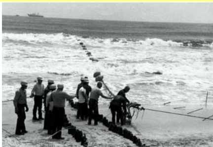
Image about the installation of a sea cable.
