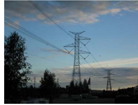
High-voltage power transmission systems are affected by geomagnetic disturbances.
